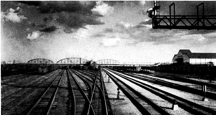
Freight yards at Winnipeg, among the largest in the world. Its central location made Winnipeg the principal rail and air centre of western Canada
